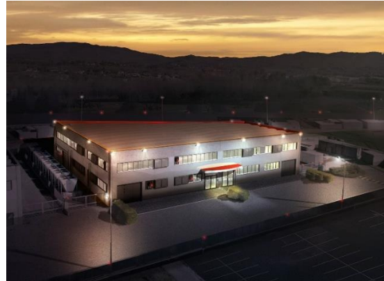
Figura 2 – Data Center IT2
