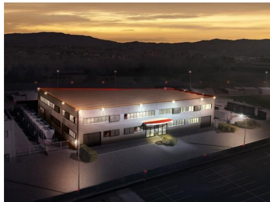
Figura 2 – Data Center IT2
